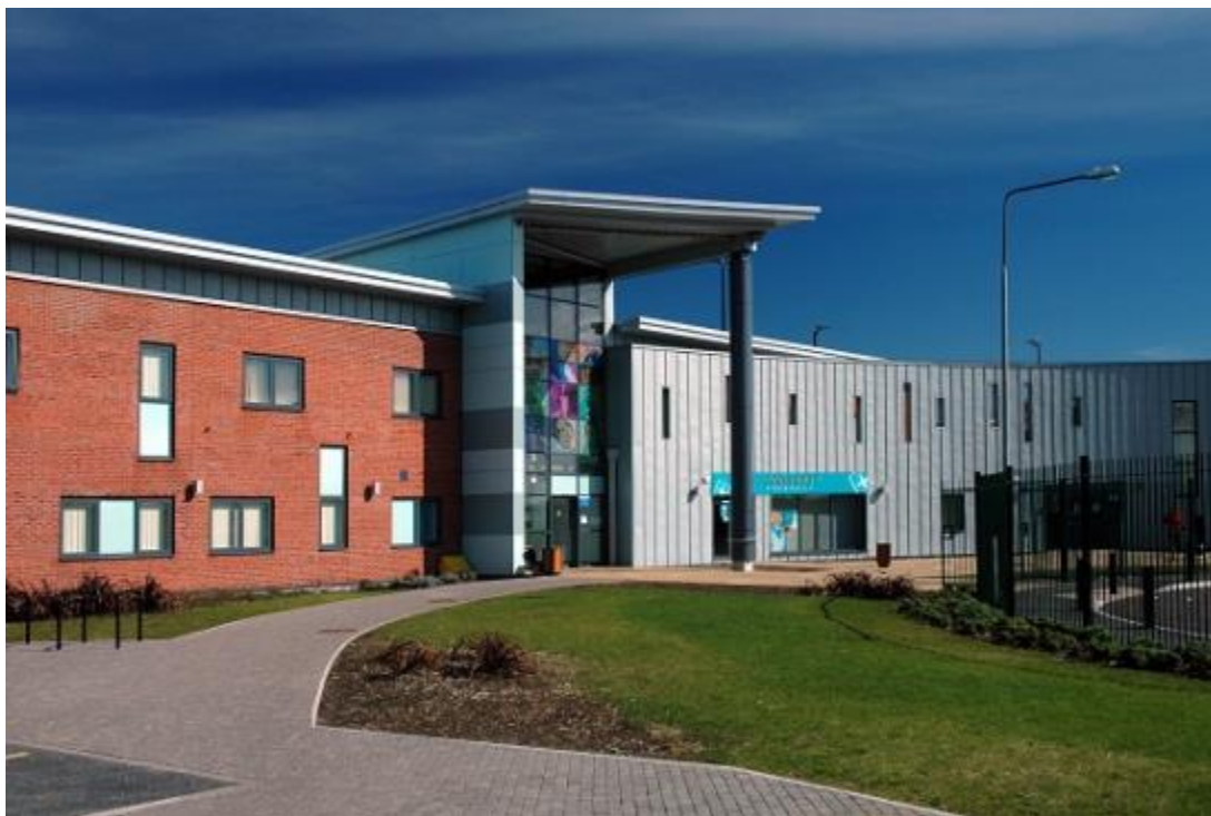
Figure 2: Dr Maassarani & Partners - Tower Hill main site
